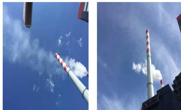
Figure 5. Plume characteristics (left: cold-side ESP, right: colder-side ESP)
