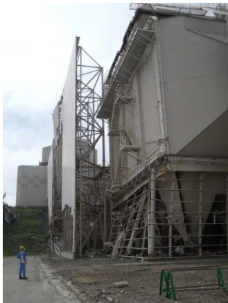
Figure 1. ESP of Haramachi Power Station Unit 1
