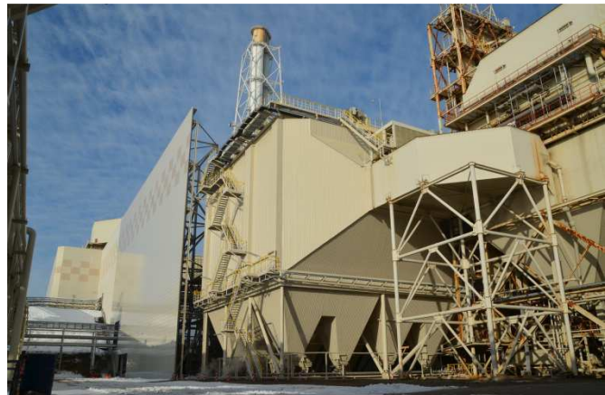
Figure 1. ESP of Haramachi Power Station Unit 1
