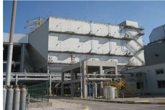
Figure 6. Outside View of MEEP installed at Coal-fired Thermal Power Station in Turkey
