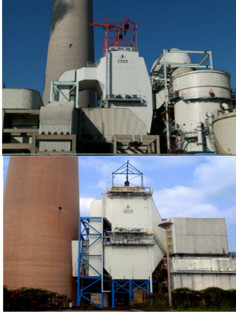
Figure 3. Wet ESPs of complex structure for 330 MW unit at Huadian Zibo power plant and for 670 MW unit at Datang Huangdao power plant
